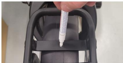
*Figure 7 - Marking the drilling hole on the mudguard.*
